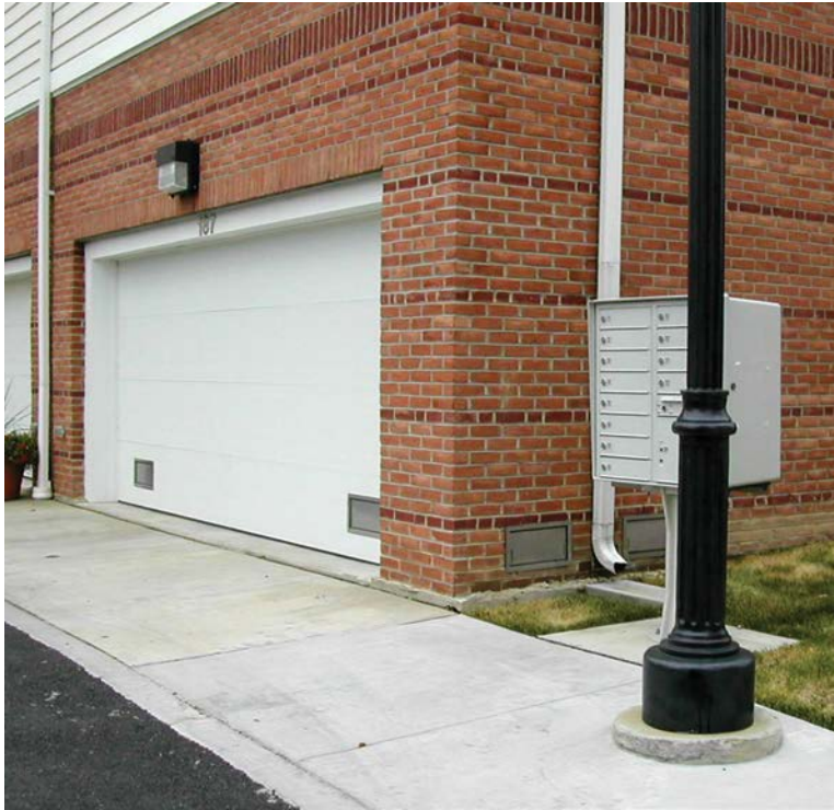
Figure 6: Engineered openings in garage doors
